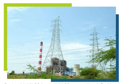
Erection of 230KV DC line on 400kV DC towers at Neyveli, Tamil Nadu, India
