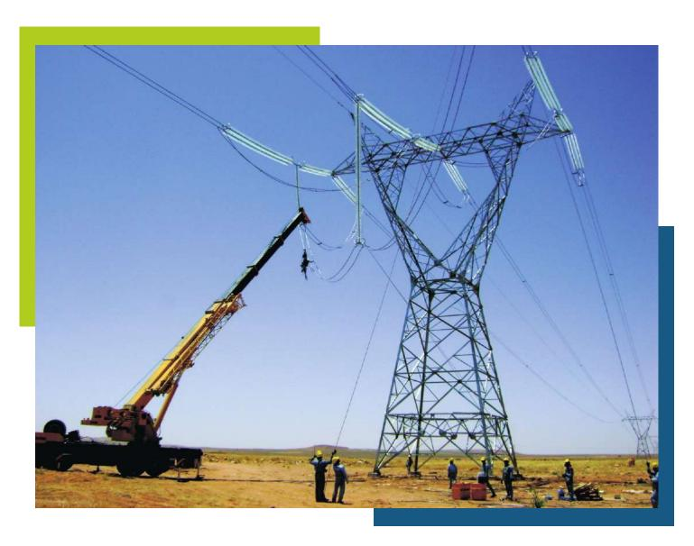
Transposing of Phases 400 KV Single Circuit Line Tilghmit, Algeria
