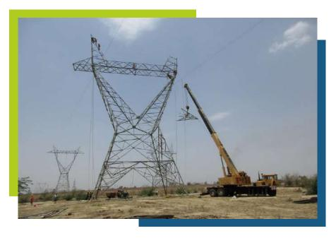
Crane Erection of 400 kV S/C Agra-Bassi Transmission Line at Bassi, India
